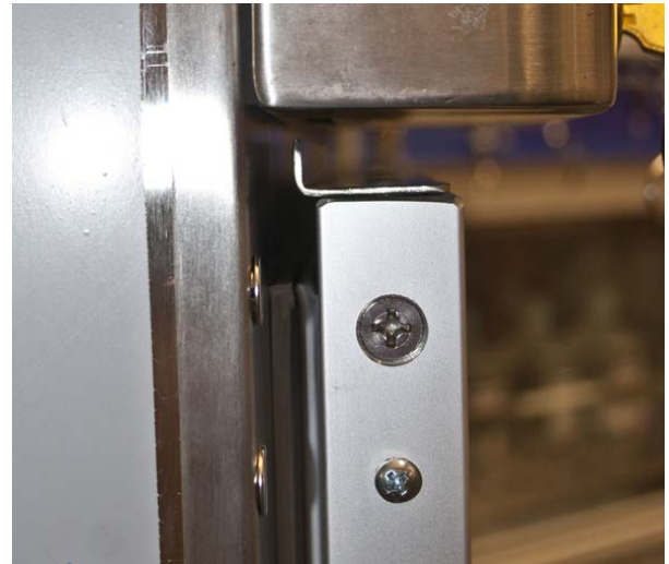
Fig. 51: Cam Lock Plate door gap
